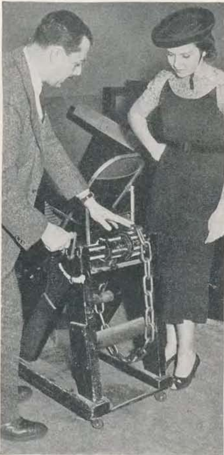
This is called a chain windlass machine. As the crank is turned, heavy chains make noises like those of a docking ship or ferry.
